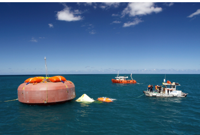
Buoyant actuators were towed offshore from Fremantle, and ballasted utilising local shore-base resources.
